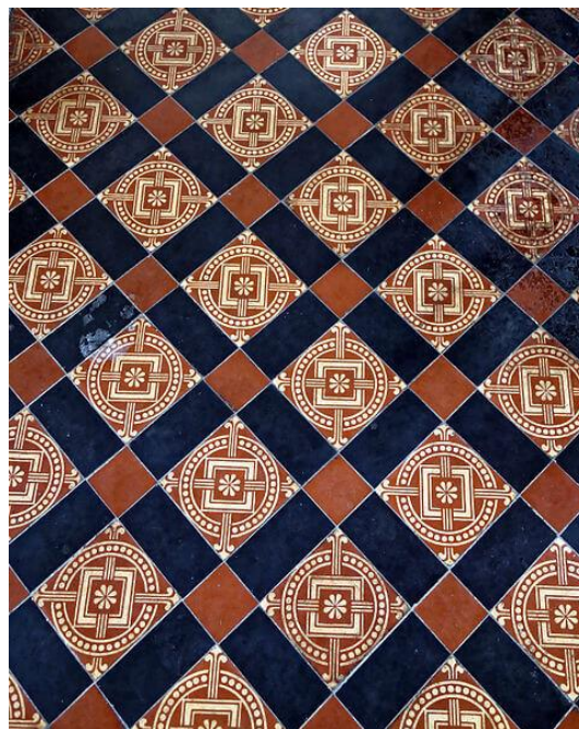
Figure 3. Encaustic Floor Tiles at St. Mary the Virgin's Church in Hatfield Broad Oak, Essex, England. Note. Image via Wikipedia Commons (Acabashi, 2015)
