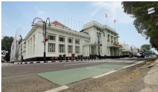
(a). Merdeka Building (the site of the 1955 Asia-Africa conference)
