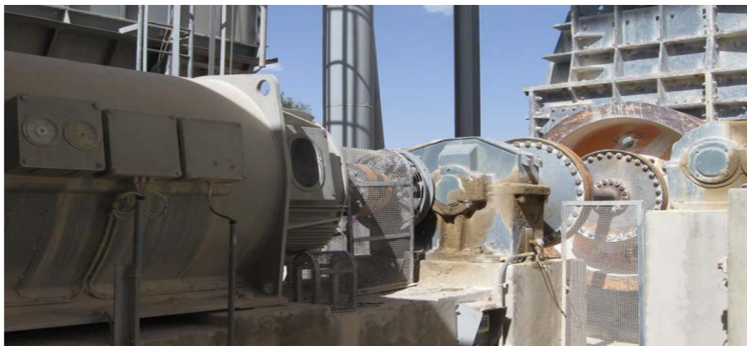
Figure 2. Crusher A1MO1 control equipment
